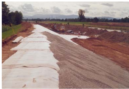
Fig. 3 Covering Bentofix® GCL with locally available fine gravel to ward off burrowing animals
