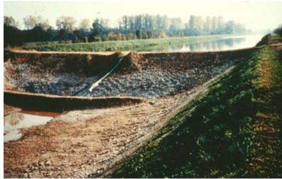
Fig. 1 Cofferdam at the Lechkanal sealed with needle-punched geosynthetics clay liner (GCL), 1989
