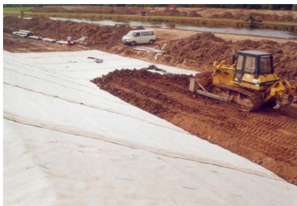
Fig. 5 Kinzig River levee reconstruction (2001)
