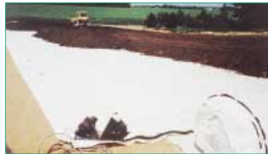
Figure 14 Secudrän® placement over a Bentofix® GCL (landfill Halle, Germany).
