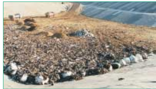
Figure 2 Filling of waste in a landfill with a Secutex® protected composite liner (landfill in Spain).
