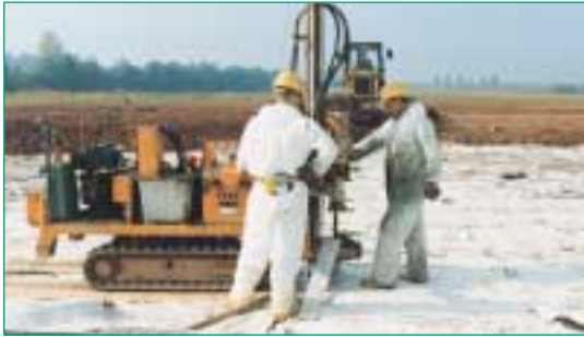
Figure 23 Installation of Secudrän® vertical drains for acceleration of consolidation.
