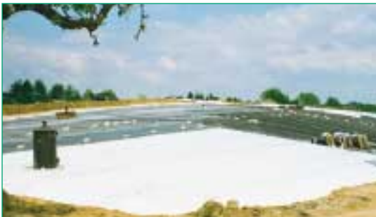
Figure 12 Composite liner with Bentofix® in a land- fill cap (landfill Bamberg, Germany).
