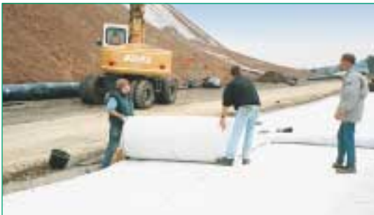
1988, shear strength transferring Secudrän® drainage systems were more widely used in landfill caps.
