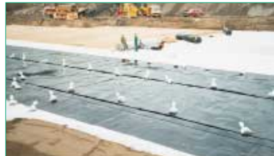
Figure 22 Carbofol® geomembrane protected between Secutex® nonwovens (business park Lammerting, Germany).
