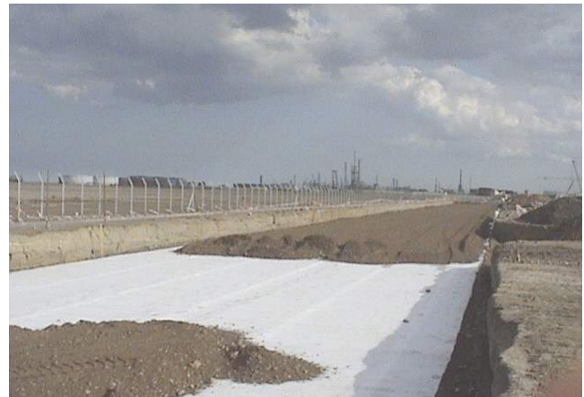
Fig. 12: Installation of Secugrid® base course reinforcement
