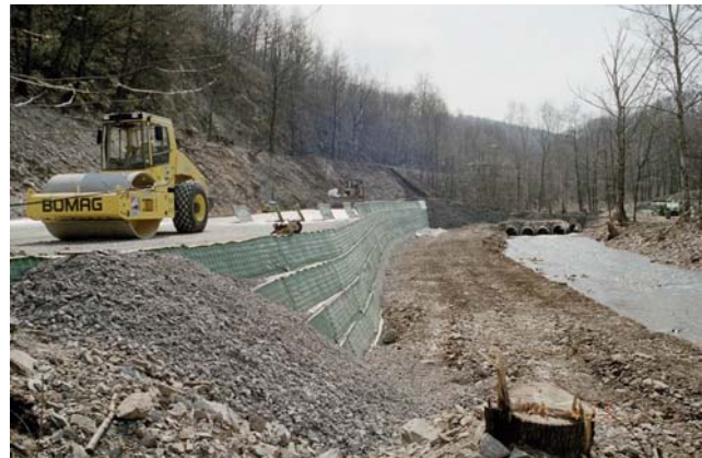
Fig. 19: Geogrid reinforced railway embankment
