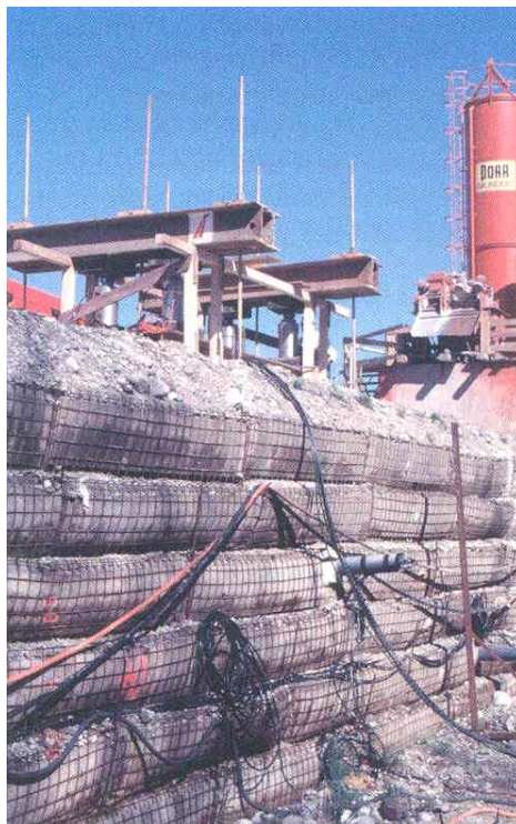
Fig. 2: Testing the bearing capacity of a geogrid reinforced soil structure.
