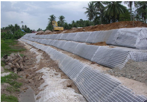
Fig. 14: Picture of reinforced slope during construction Fig. 15: Picture of finished project
