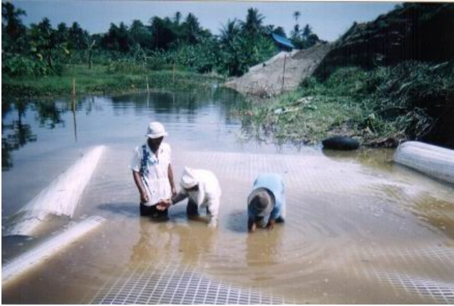
Fig. 13: Extreme soil conditions on site
