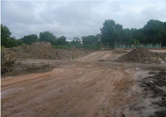
Fig. 16. Existing site conditions
