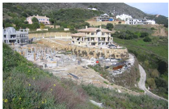
Fig. 25: Constructed villa on reinforced soil structure (May 2006)
