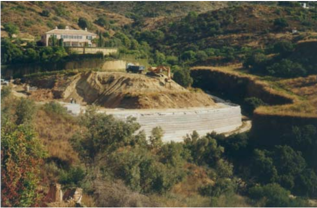
Fig. 22: Construction of the base wall (10 m high)
