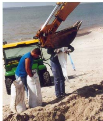
Photo 7 Filling Geotextile Bag
