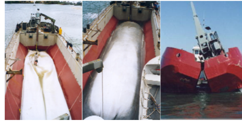
Photo 5 Geotextile Container in Barge
