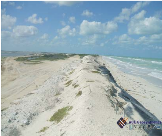
Photo 1 Geotextile Back Beach Protection.
