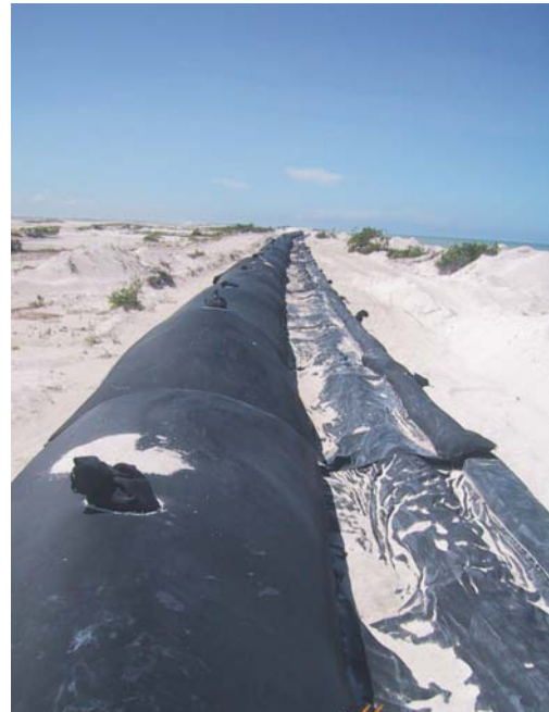
Photo 3 Geotextile with Scour Apron
