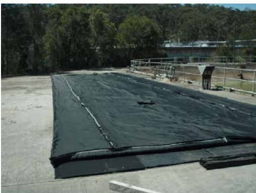
Photo 8 Positioning the geotextile tube.
