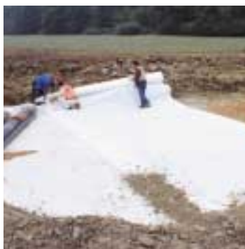
Installation of Combigrid® as stabilisation on the Cremlingen B1 bypass, Germany
