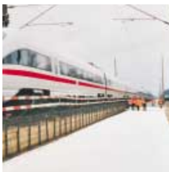
Combigrid® in use under the railway line at Hagenow, Germany
