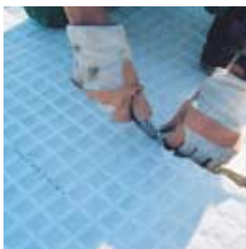
Cutting Combigrid® to size using commercially available tools
