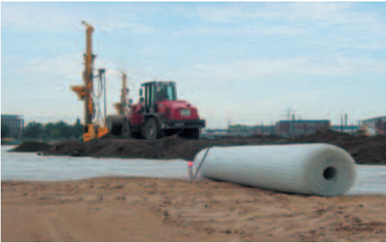
Unrolling of Secugrid®
