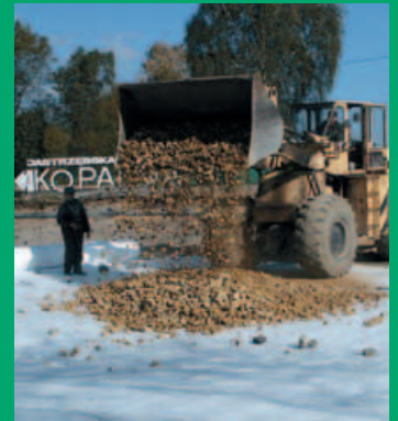
Fig. 5 Placing crushed aggregate on Secugrid®
