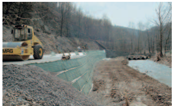
Compaction of fill aggregate
