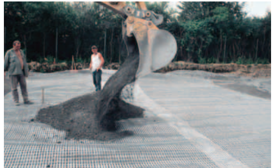
Cover soil placement
