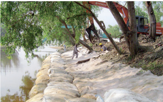
Placed Terrafix Soft Rock® prior to soil coverage
