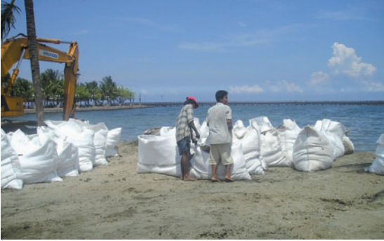
Filled Soft Rock prior to closure
