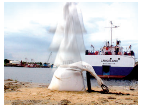
Fig. 3 Terrafix Soft Rock® container in a dropping installation performance
