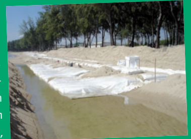
Fig. 6 Soft Rock Containers on site and ready to be filled
