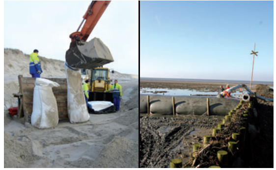
Filling of Soft Rock containers
