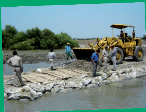
Fig. 5 Placement of cover material over the Terrafix Soft Rock® jetty
