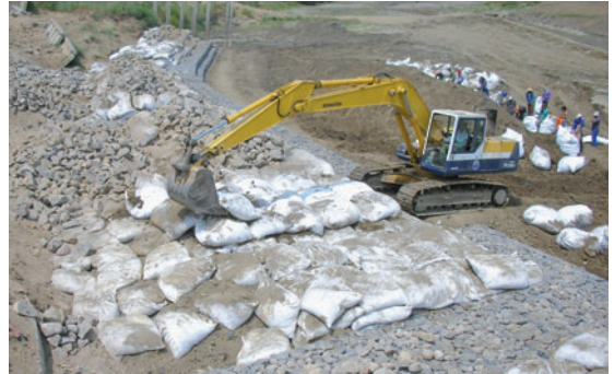
Placement of Terrafix Soft Rock®
