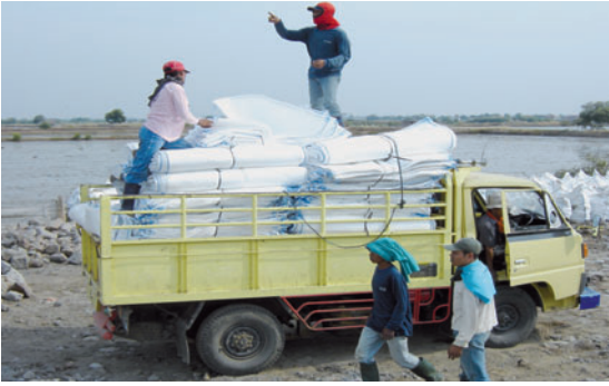
Terrafix Soft Rock® delivery on site
