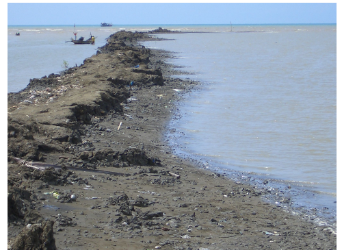
Overview old Jetty
