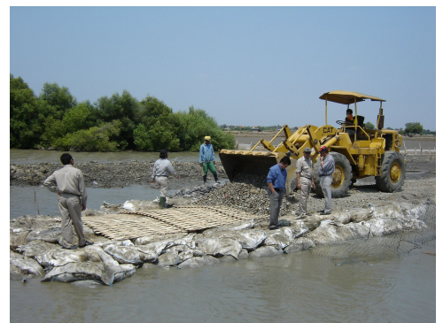
Inspection during the installation
