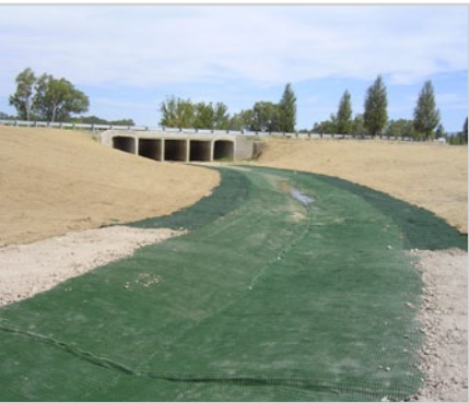
FIG.1: PYRAMAT & LANDLOK 450 INSTALLED
