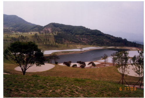
View over the project
