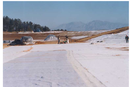
Installation of Bentofix®
