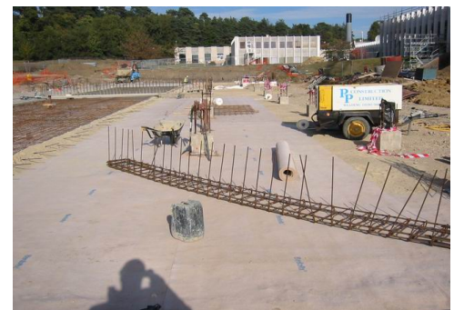
Bentofix® BFG 5000 as basement waterproofing
