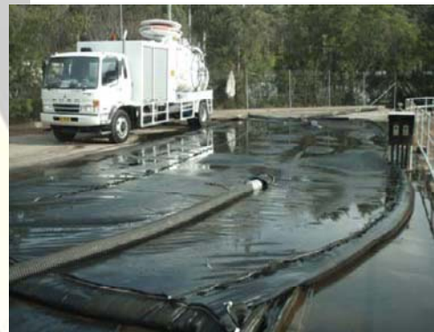
Filling of geotextile tube commences
