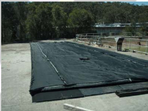
Positioning the geotextile tube
