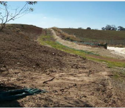
FIG.4: VIEW OF CHANNEL
