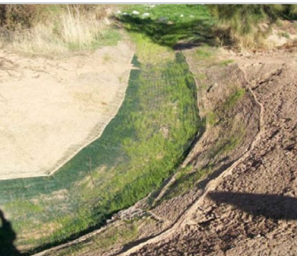
FIG.5: VIEW OF CHANNEL
