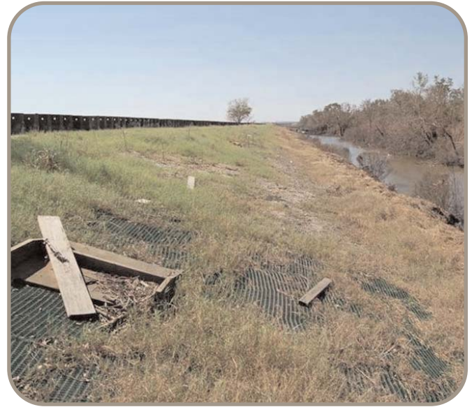
ArmorMax System Withstands Debris Loading from IKE
