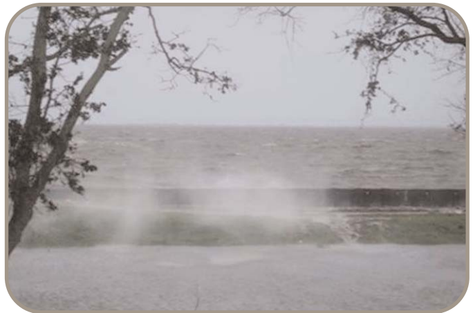
Hurricane IKE Storm Surge at 6:22 pm
