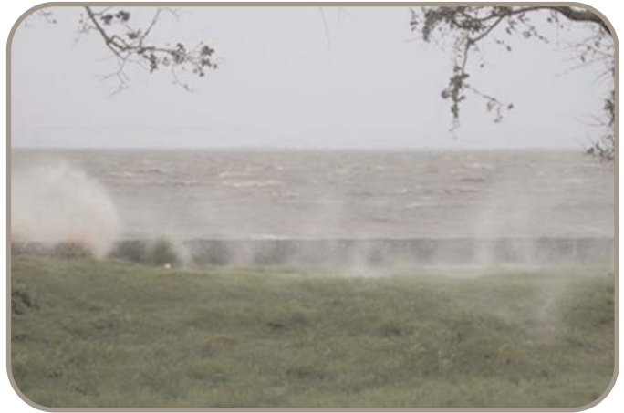
Hurricane IKE Storm Surge at 3:17 pm
