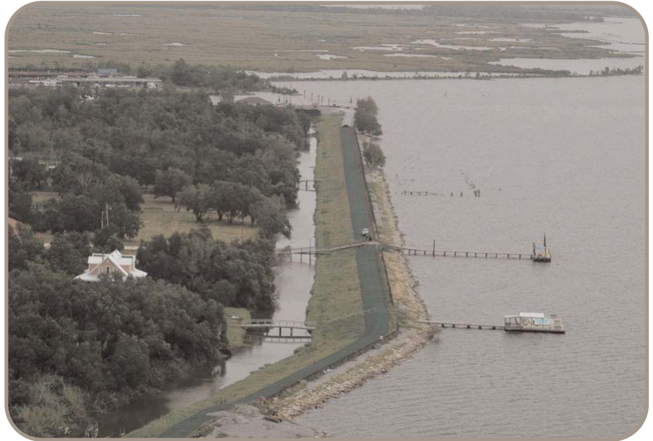
Penn Levee Phase I installation completed summer of 2007
