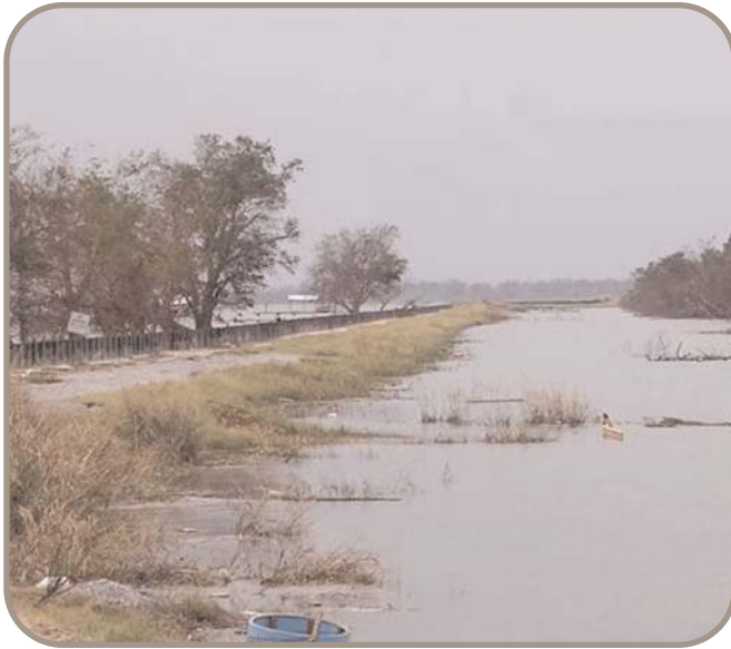
Three Days After IKE Storm Surge & Flooding
