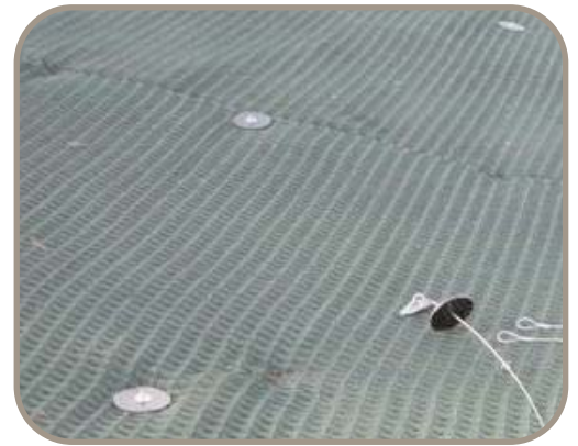
ArmorMax® System consists of HPTRM and earth percussion anchors
