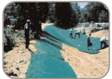
June, 1995 Installation of Landlok® TRM 450
