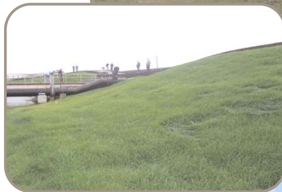
February 2007: ArmorMax™ protected slope after 9 weeks vegetation.
