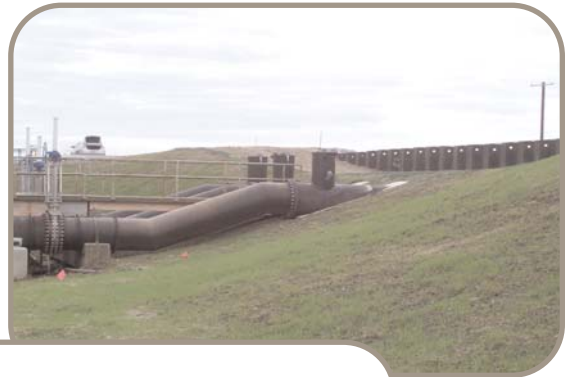
January 2007: ArmorMax™ protected slope after 4 weeks vegetation.
