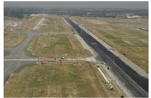
Runway widening with Bentofix® for environmental protection
