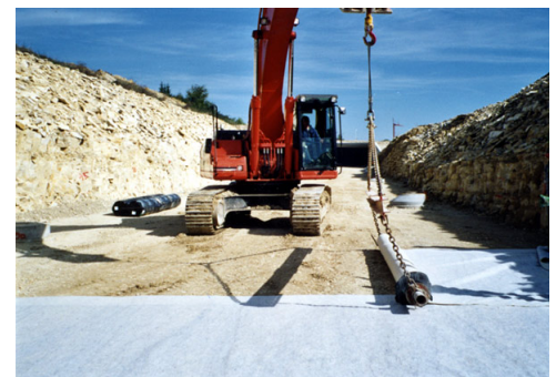
Installation of Bentofix®
