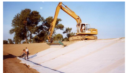
Installing Bentofix® sealing to the water-side
