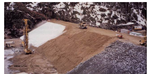
Soil placement on Bentofix®
