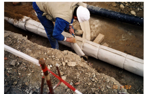
Attaching Bentofix® to the sewage line
